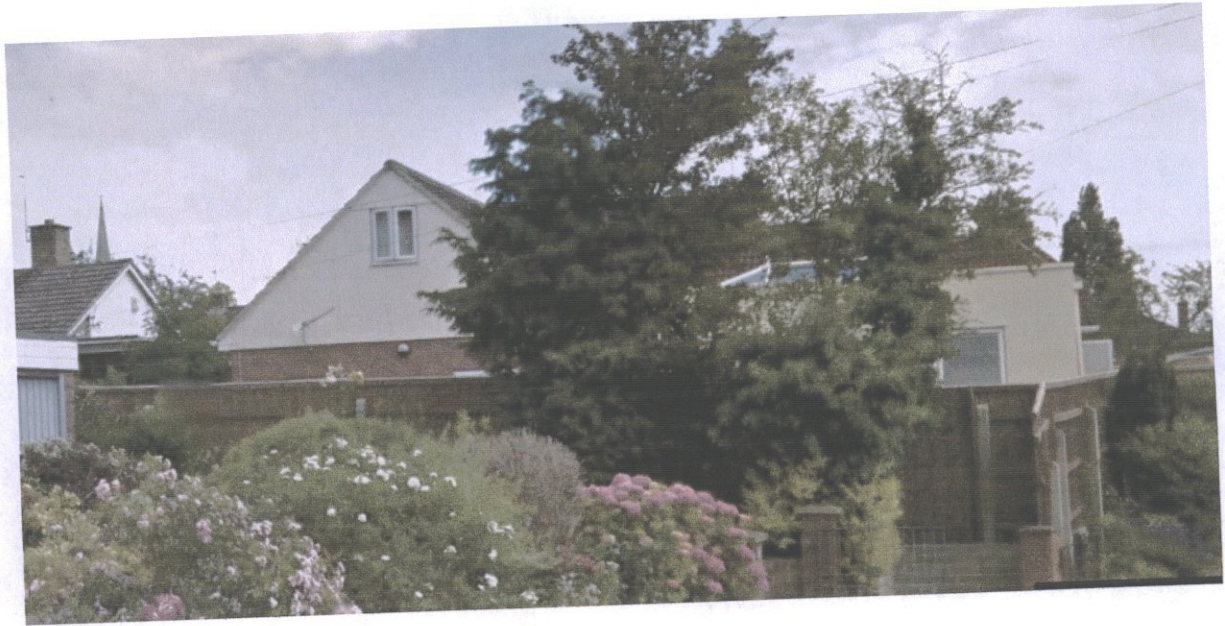
Photograph 7, rear elevation of Morelands taken from Milton Avenue, The Acorns is to the left
